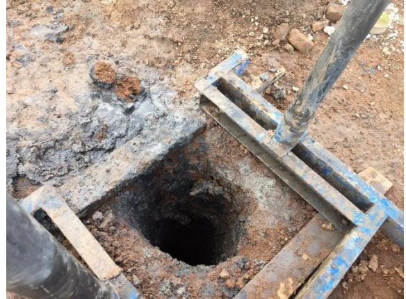
Gambar 8. Lubang Pondasi Strauss Pile
