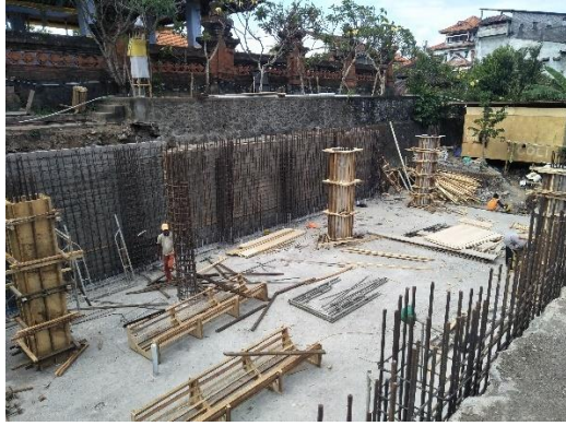
Gambar 9. Pembesian Retaining Wall
